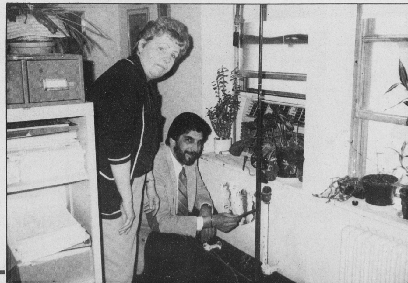
FAST ACTION — CSEA Nassau County Local 830 Safety and Health Committee chairperson John Aloisio and Alcohol and Drug Rehabilitation Unit President Adelle Rosamelia inspect a freshly sealed wall in a building at Nassau County Medical Center where asbestos was identified during CSEA's safety sweep. The administration immediately acted to seal up the wall after CSEA brought the potential danger to their attention.
