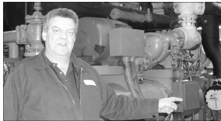
Refrigeration Plant Supervisor Tom Borden points to the compressors used to cool the ice rinks at the Olympic Complex, the site of the U.S. hockey team's "Miracle on Ice" defeat of the Soviet hockey team.
