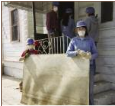
These Circle K members spent part of their winter break in New Orleans, gutting homes damaged by Hurricane Katrina in 2005.
