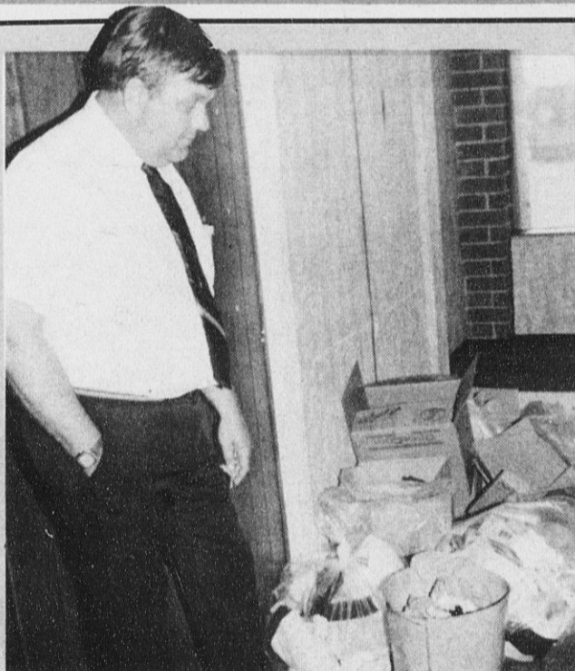
GARBAGE GALORE — CSEA Occupational Safety and Health Specialist Ken Brotherton notes trash piled on second floor of Suffolk County Department of Social Services Babylon Center. The cleaning contractor refused to remove the trash since the elevator is shut down.
