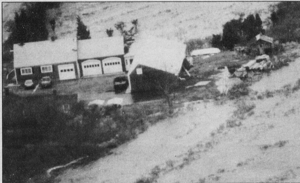
Orient Point Park's office surrounded by water after the December 1992 Nor'easter.
