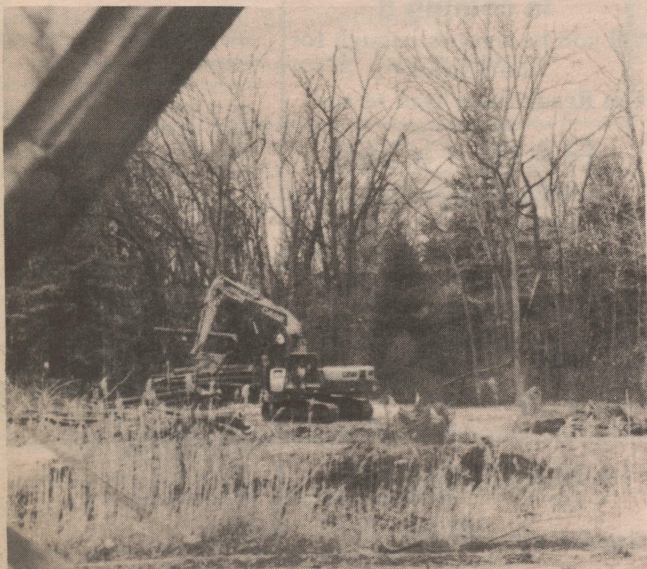
The SUNYA fieldhouse is under construction and will be completed in 1991.
