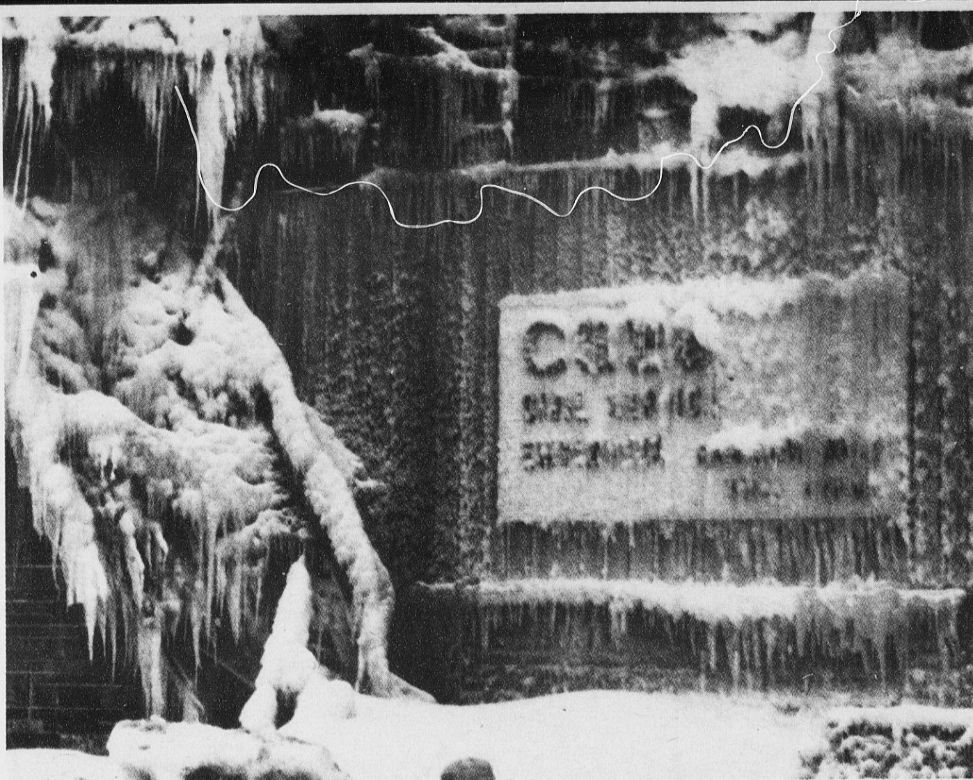
BENEATH A THICK LAYER OF ICE , the words "CSEA Civil Service Employees Association" are barely visible in the aftermath of a fire which destroyed the building housing the Utica offices of the union.
