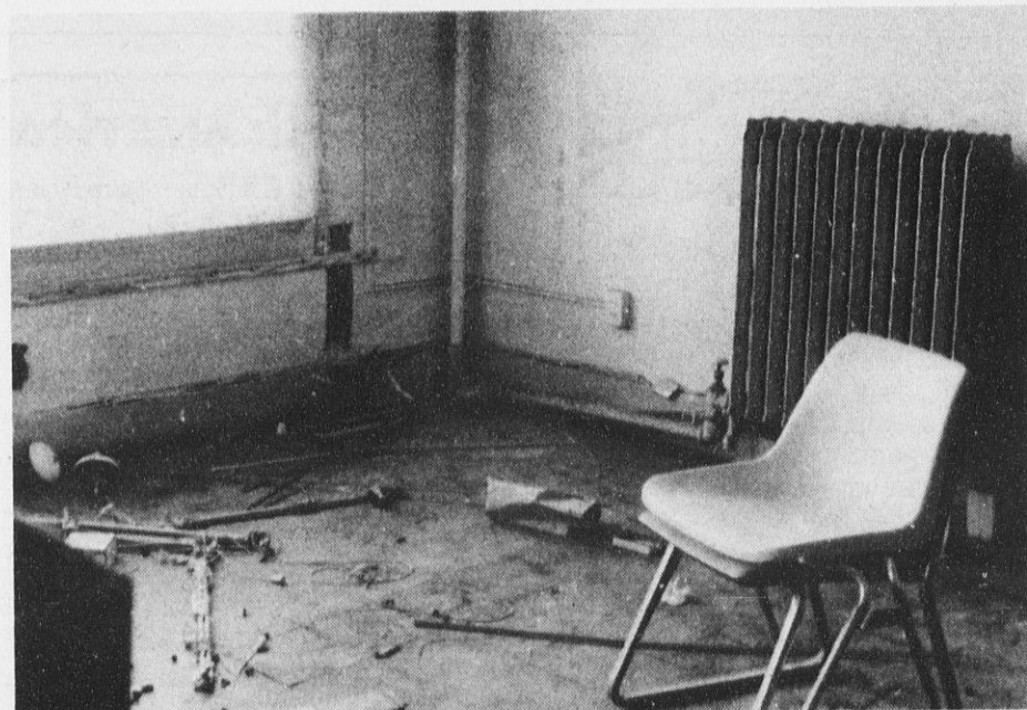
SOMETHING OLD — A picture of the old Dutchess County Courthouse annex before renovations by the Department of Public Works crew members.
