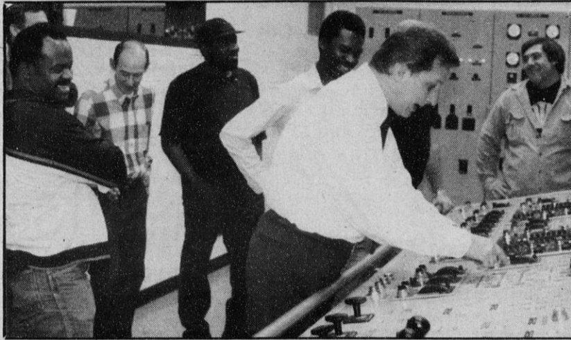
CSEA-REPRESENTED stationary engineers sharpened their skills on handling boiler emergencies at a seminar sponsored by the Joint CSEA-NYS Labor Management Committees. The seminars were held at LaGuardia Airport, Queens, after two major emergencies at Creedmoor and Kingboro psychiatric centers.
