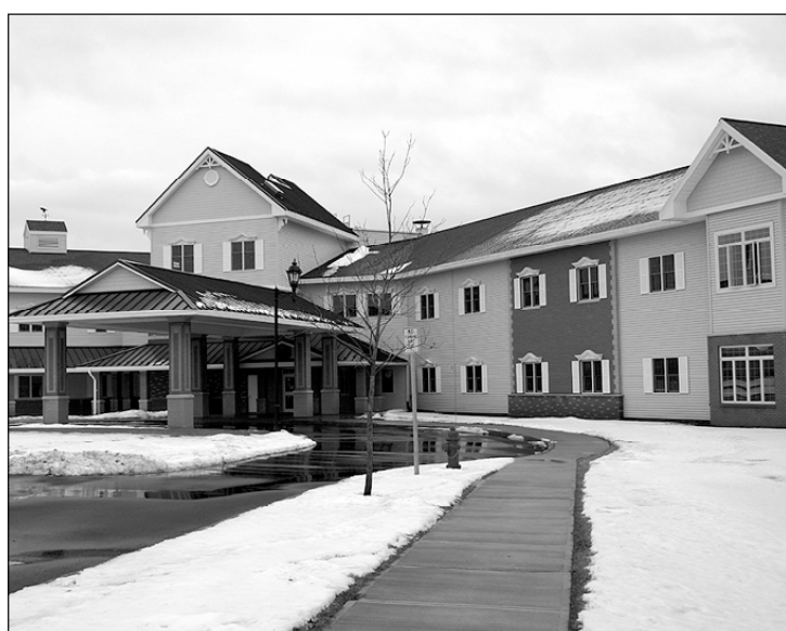
Outside view of the Otsego Manor nursing home. By building a new nursing home, the county is receiving more funding, cutting costs so the move also keeps the nursing home public, under county ownership.
