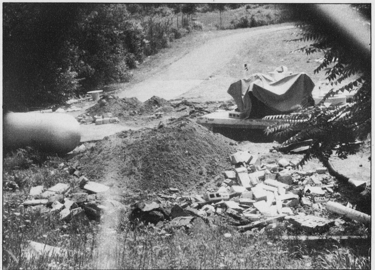
THE REMAINS OF THE COHOES PUMPING STATION lay scattered all around the worksite after the explosion which injured two CSEA members. The cause of the explosion may have been from a propane gas leak — the cylinder at the left is a large propane tank.
