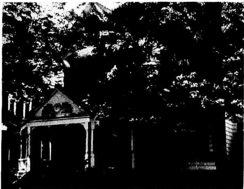
The new Alpha Pi Alpha fraternity house is located at 135 South Lake Avenue. At present, twenty men are living there. When renovations are complete, the house will accommodate over thirty of the brothers.
