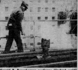
Harold P. Rosenberger performs "instant weld" on third rail while the power is maintained on the rail to insure non-interruption of service during repairs.
