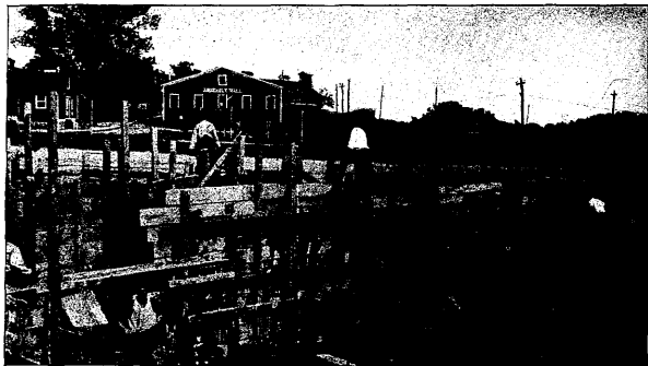
Administration Building Under Construction, New Hampton Farms.
