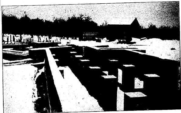
Foundation of Administration Building, New Hampton Farms.
