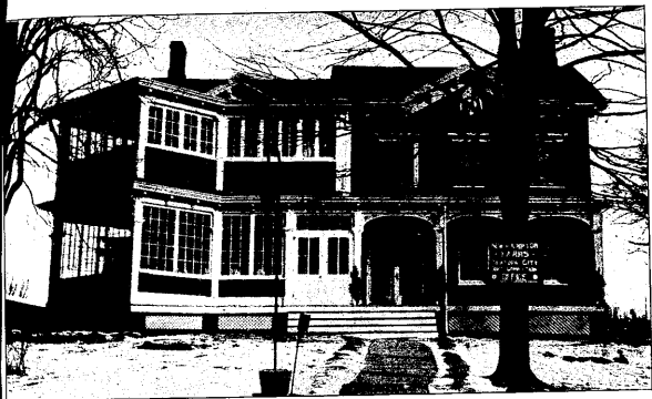
Superintendent's Residence, New Hampton Farms.
