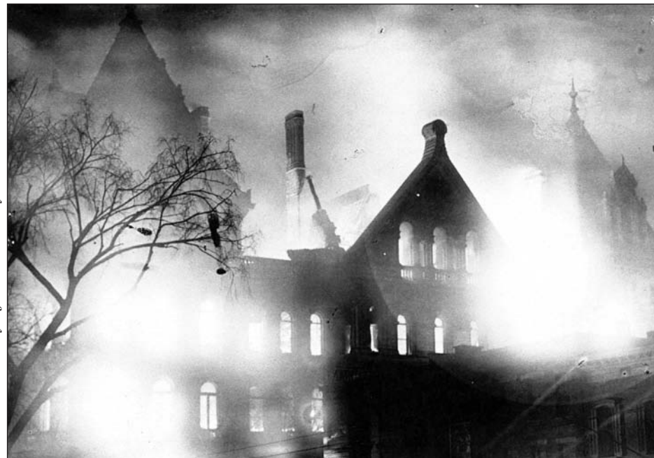
New York State Capitol engulfed in flames the evening of March 29, 1911.
