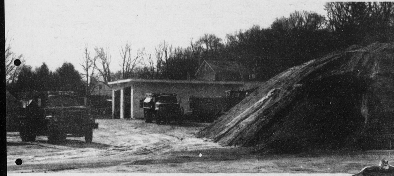
RAIN turns the unpaved yard at the DOT Katonah facility into a muddy quagmire. The doorless building in the rear of the yard is where vehicle maintenance and repairs are carried out year round.
