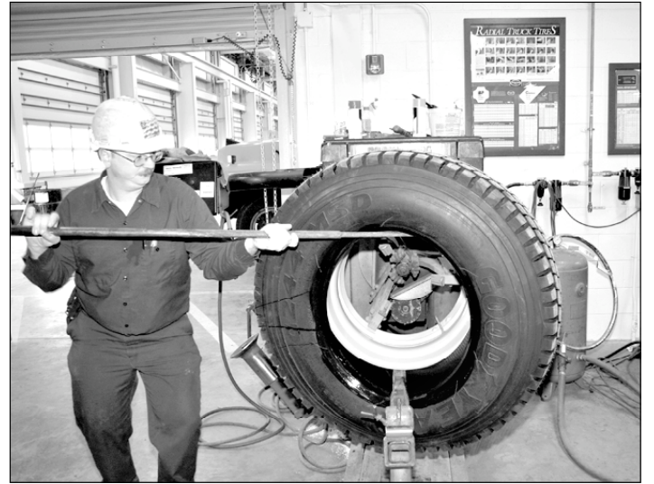
CSEA tire service mechanic Tim Bloodgood mounts a tire on a rim, which previously had to be done at a facility miles away.
