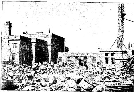
Prison Farm, Guelph, Ont. Building under Construction by Prison Labor.
