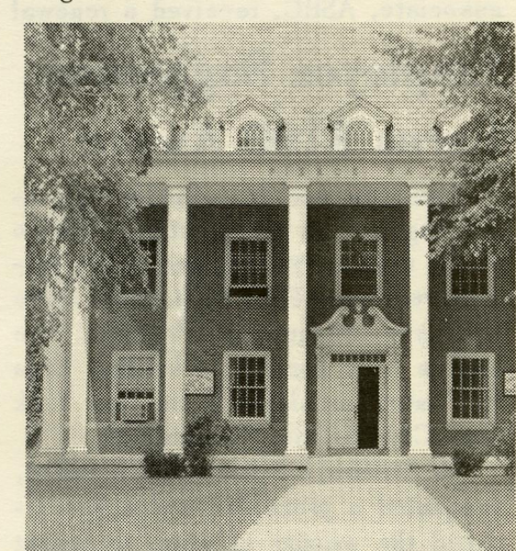
THE STately FACADE of Pierce Hall will once again greet resident students when school opens in the fall.
