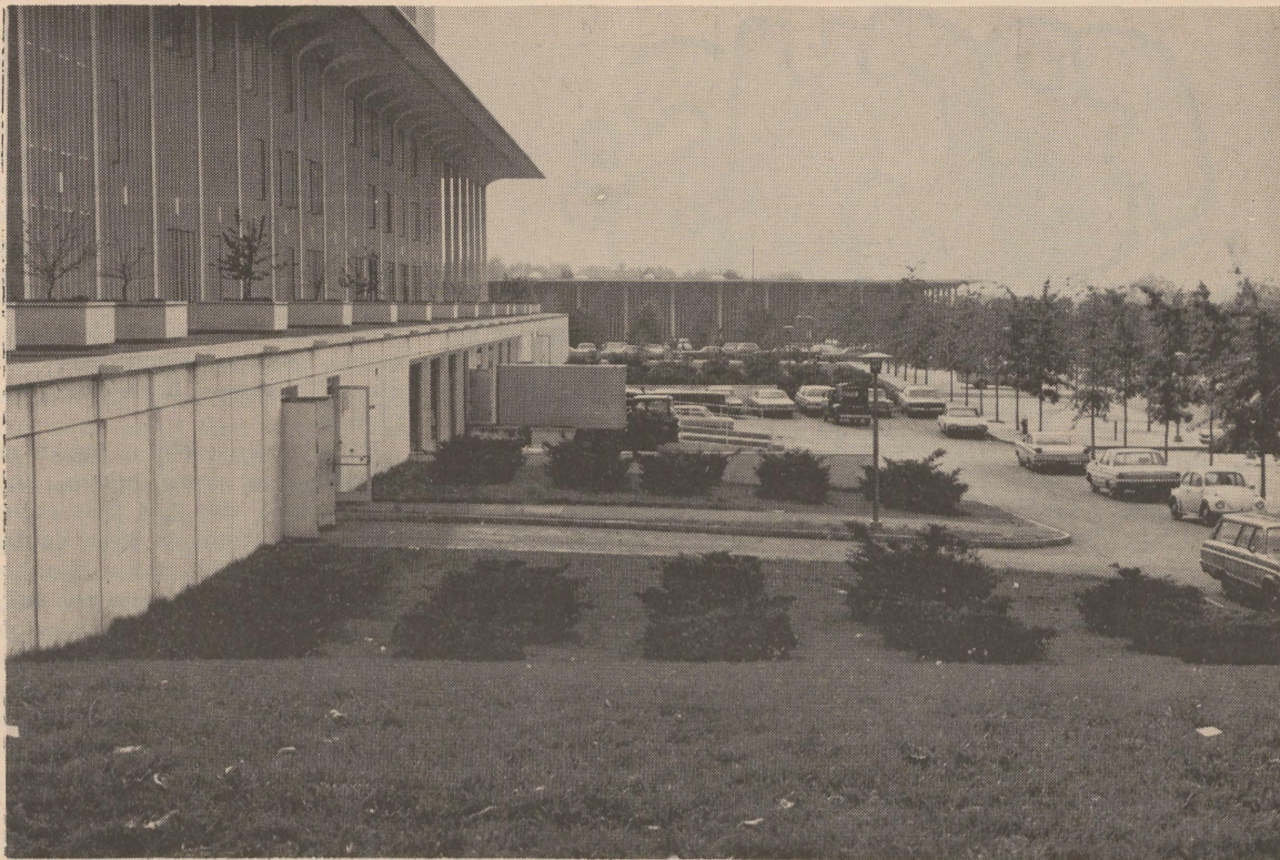
The site of the proposed west podium extension.
