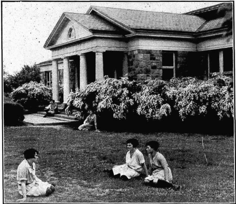
ONE OF ATTRACTIVE BUILDINGS AT LETCHWORTH
