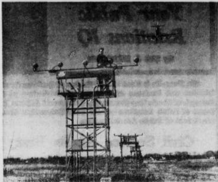
Checking Emergency Lighting
