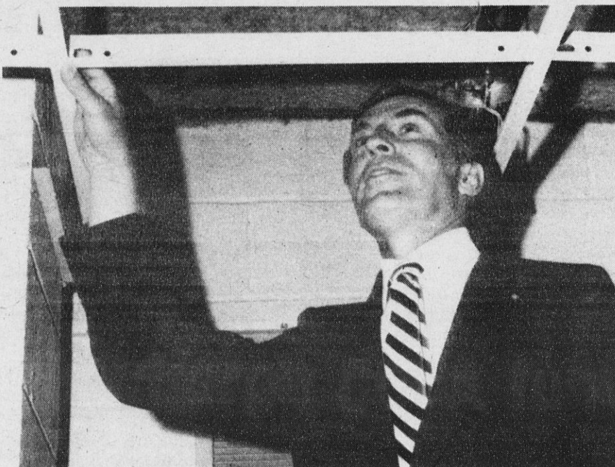
NEW ROCHELLE MAYOR Leonard C. Paduano inspects the newly constructed frame for the drop ceiling of the City Hall storeroom. The ceiling above is insulated with a material containing asbestos which has been flaking off and falling.
