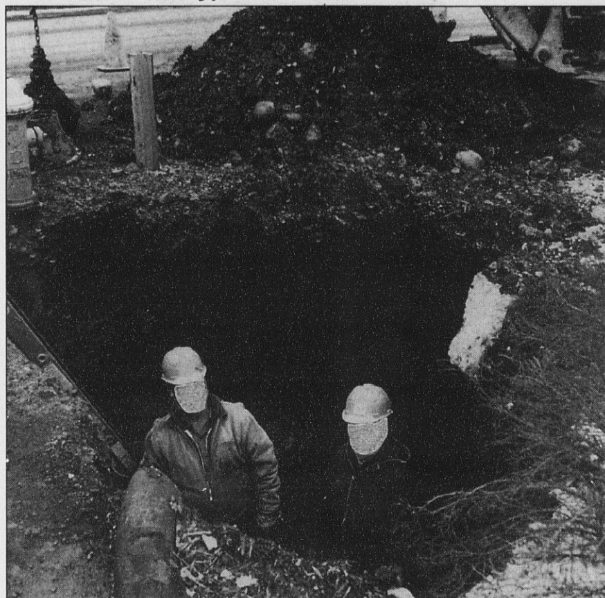
These unidentified CSEA members have placed themselves in very real danger. The pit they have dug has no shoring.
