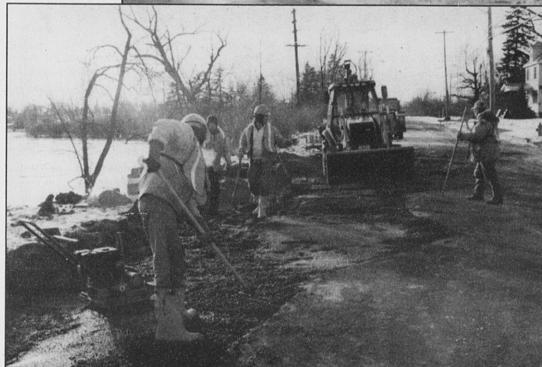
CSEA CITY OF WATERTOWN DPW UNIT members shore up and patch section of Water Street that was damaged by ice and flooding.
