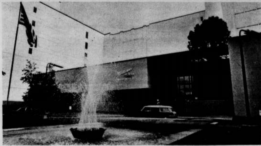
Drive up to Midtown Plaza at 700 East Water St. in Syracuse, home office of the CSEA Syracuse Region. Well-manicured greenery and a spraying fountain generate a pastoral illusion in mid-city.
