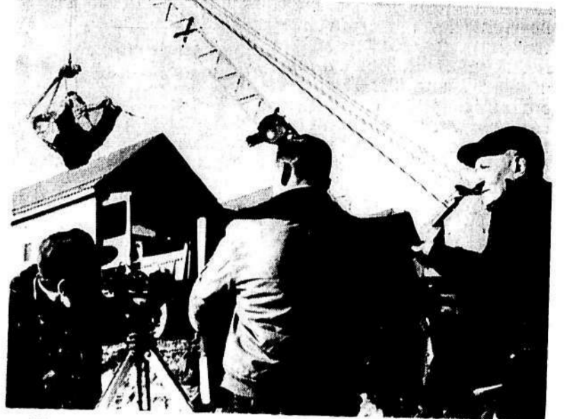
Above, construction workers on State's new Western Avenue dormitory pose with the implements of their trade for NEWS photographer, Willard Gillette.
