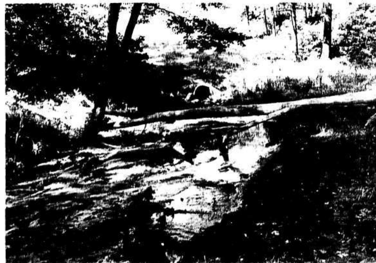
Erosion has filled in part of the pond and caused trees to fall. Drainage pipes deposit water and oil in the pond.
