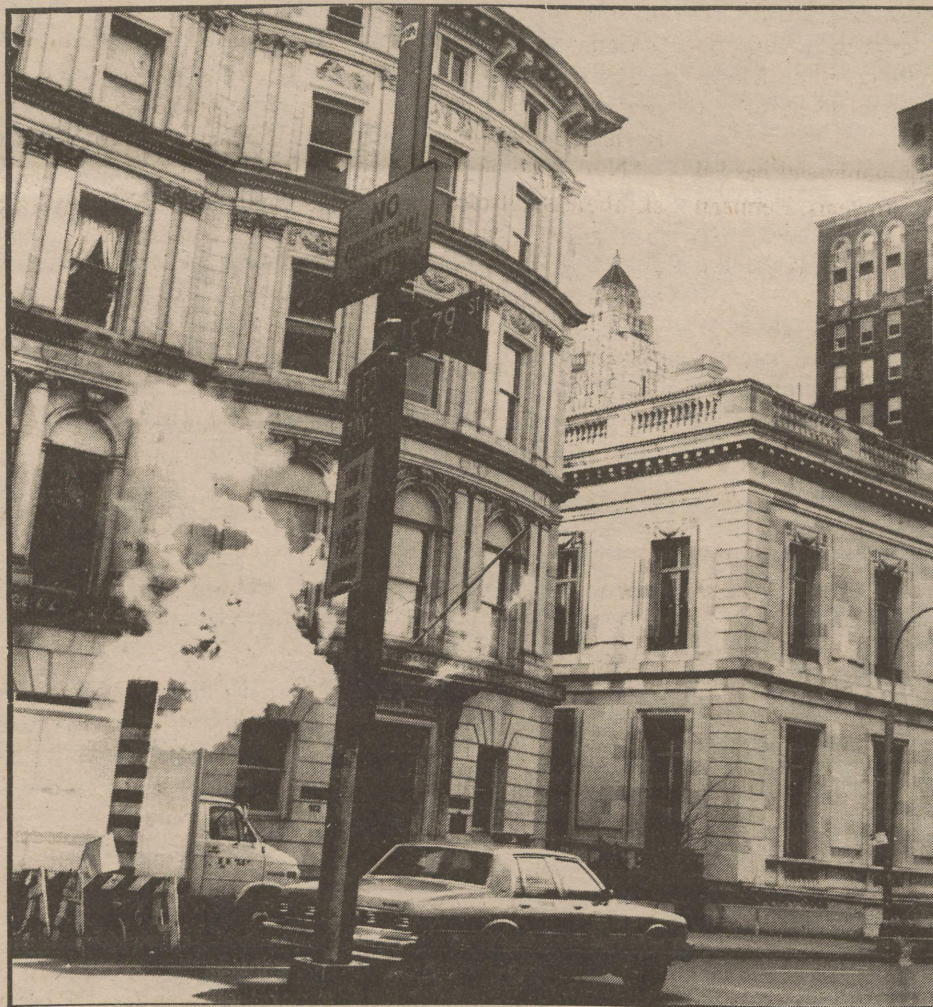
Is the building really leaning?
