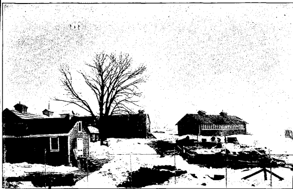
New Hampton Farms. Construction Camp.
