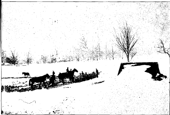
Excavating by Inmate Labor. New Hampton Farms.
