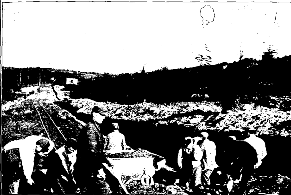
New Hampton Farms. Building Railroad Spur.
