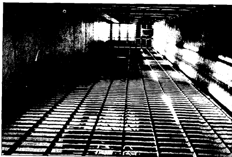
The Exercise Corridor in an "All-Steel, Inside-Cell" County Jail.
