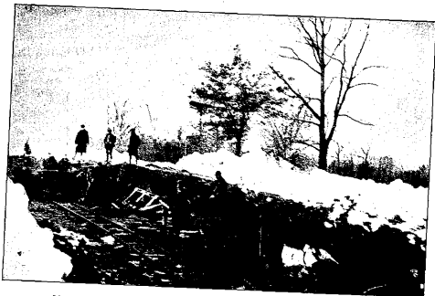
New Hampton Farms. Building Railroad Spur by Inmate Labor.
