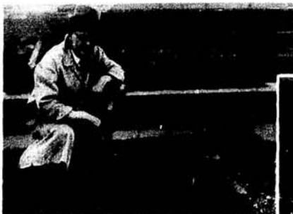
A CEMETERY WITHOUT CORPSES has been established by Prof. R. L. Dowdell of the University of Minnesota. To test the effect of soil corrosion, he has buried 1,000 pieces of metal used in funeral merchandise. Here are two views of his experiment.
