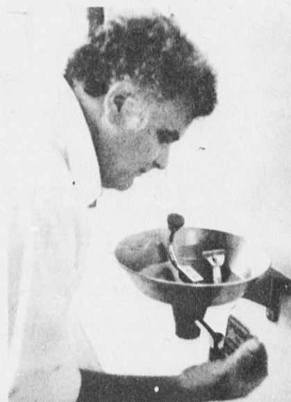
PLANT OPERATOR TOM CONROY prepares to show off one of several special eyewashes which have been installed as an extra health precaution.
