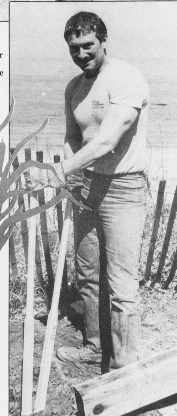
JOHN DIMARTINI rebuilds fences at Caumsett Park in Huntington.
