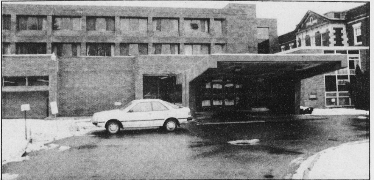
ENTRANCE to Greene County Memorial Hospital. More than half of Greene County employees work here and the county in nursing home, and their status is in doubt after Dec. 31. The facility will be operated by a private sector hospital effective that date, but CSEA contends a six-month transition period agreement covering the employees is not being honored by county officials. Meanwhile, union members have ratified a tentative four-year contract covering all employees.
