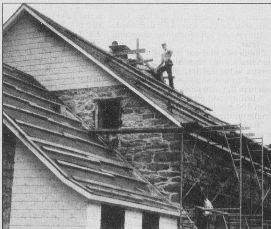
CSEA members work on historic house at Ulster Correctional Facility.
