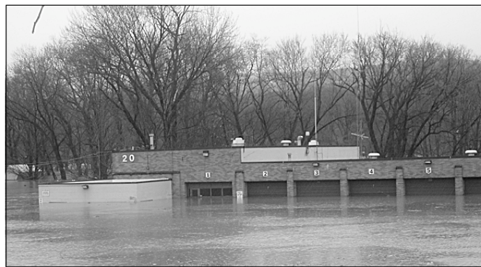
Above, the Port Jervis School District Transportation garage falls victim to devastating floods. (Photo by Betty Lou Kranz.)
