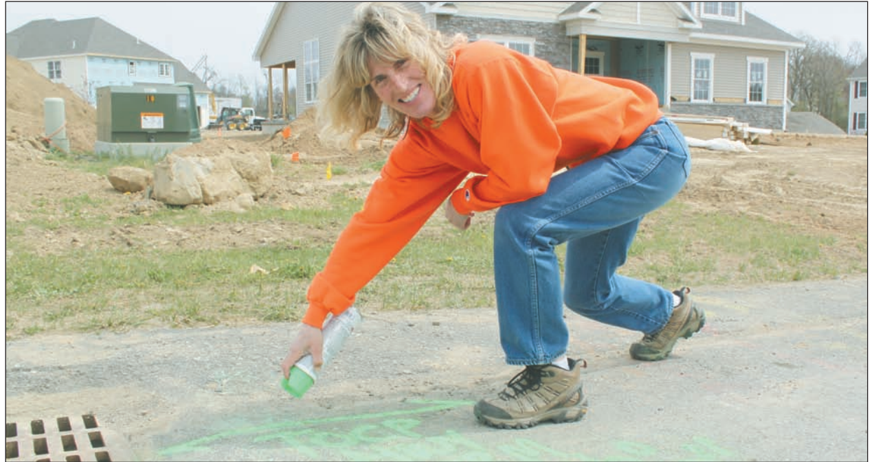
Lori Miller marks sewer lines at a Clifton Park building project.
