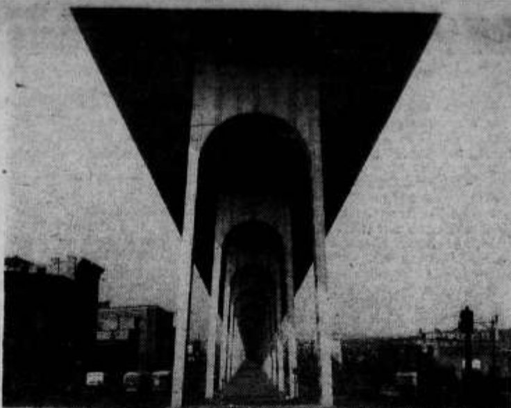
Routes through cities present one of the knottiest of all traffic problems. This is Gowanus Elevated Parkway, showing 10 lanes of service road traffic on street level with elevated structure supporting six lanes of express traffic. "Cantilever" construction allows more light and air for street below.
