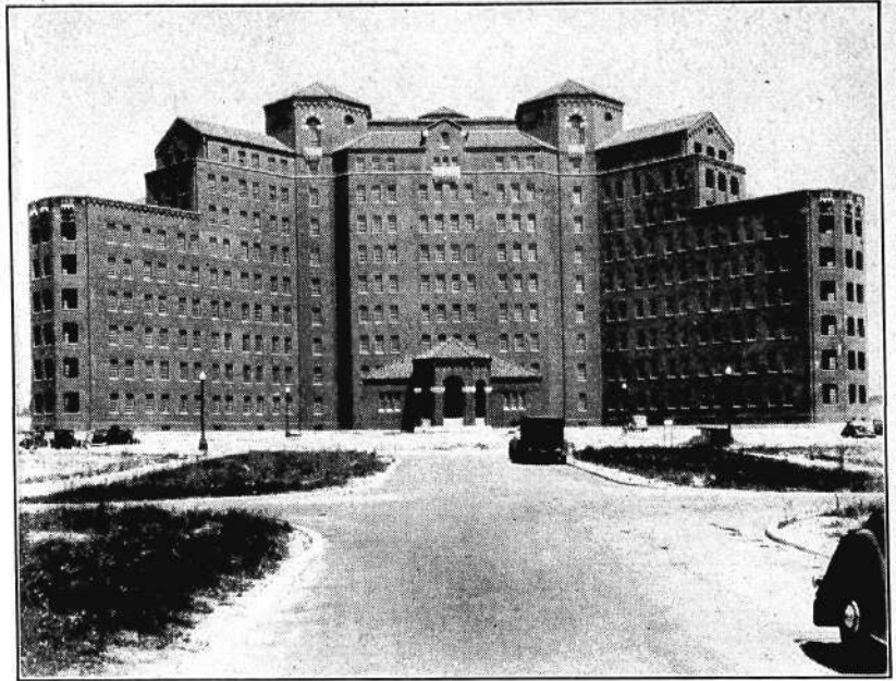
Building for feeble and infirm patients at Pilgrim State Hospital, Brentwood, Long Island. This multi-story building represents the type of construction now used for infirm patients.
