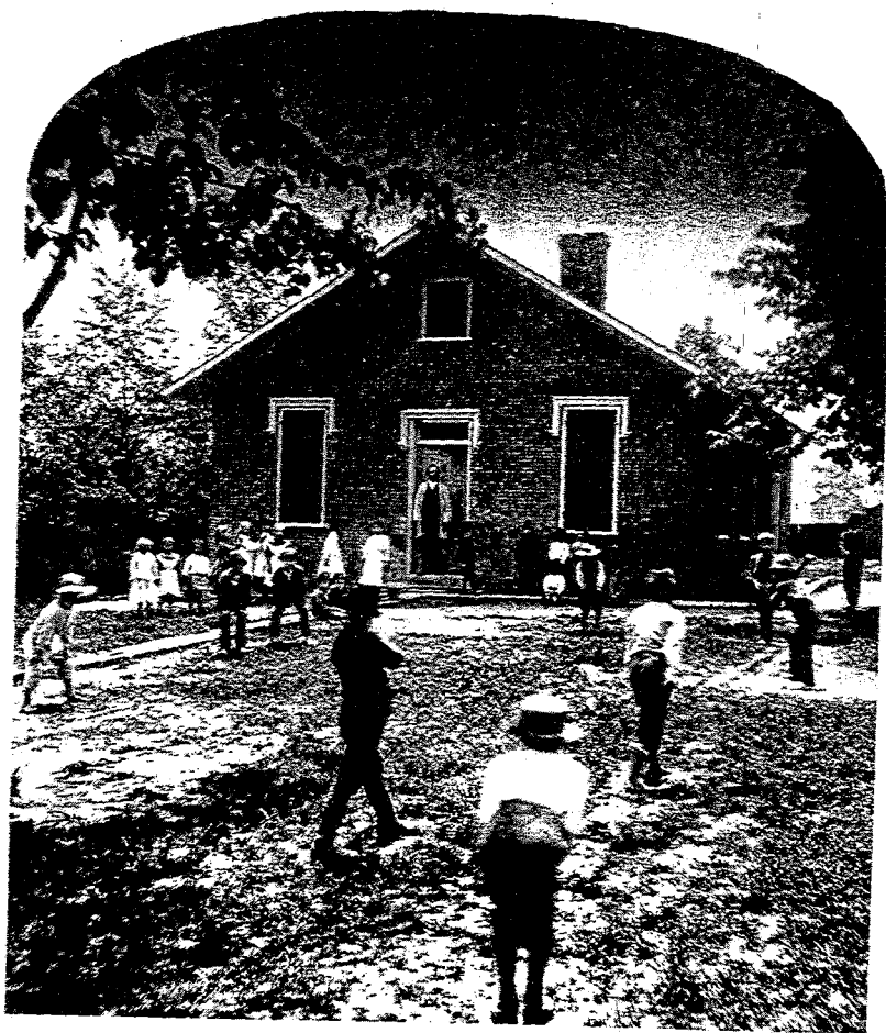
The Colored Public School of Geneva, New York, occupied this building from 1853, when the building was built, to 1873, when the colored school was abolished. Courtesy of The New-York Historical Society, New York City.
