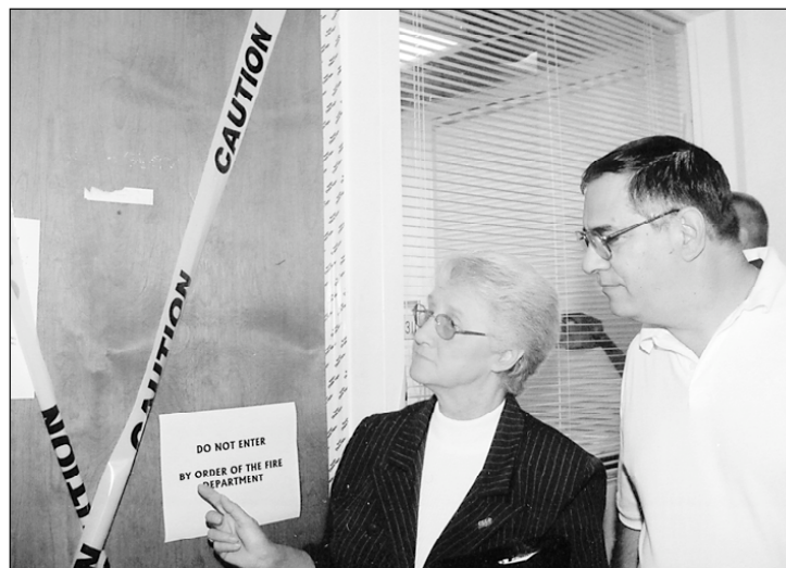
CSEA Southern Region President Diane Hewitt and Rockland County Local President William Riccaldo inspect area of leak that forced Rockland County Medical Center evacuation.
