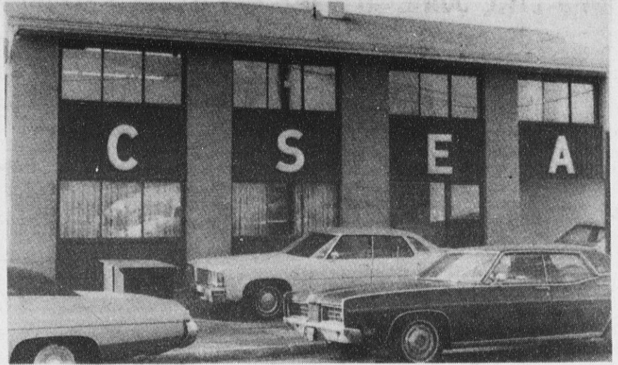
THE HUB OF CSEA ACTIVITY IN LONG ISLAND REGION I is the regional headquarters at 740 Broadway in North Amityville. From the two-story building which proudly displays the letters CSEA, the union's activities in Nassau and Suffolk counties are directed.
