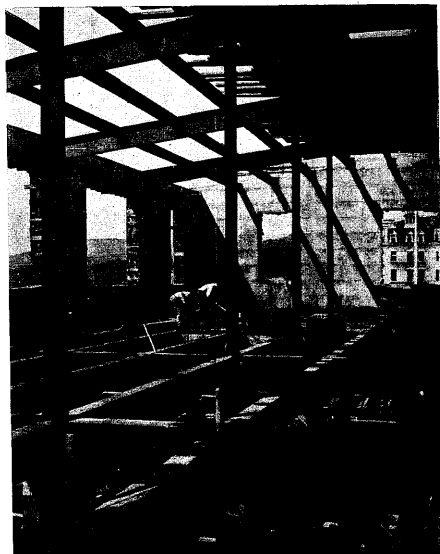
Construction — factory building — by inmate labor, Clinton Prison.
