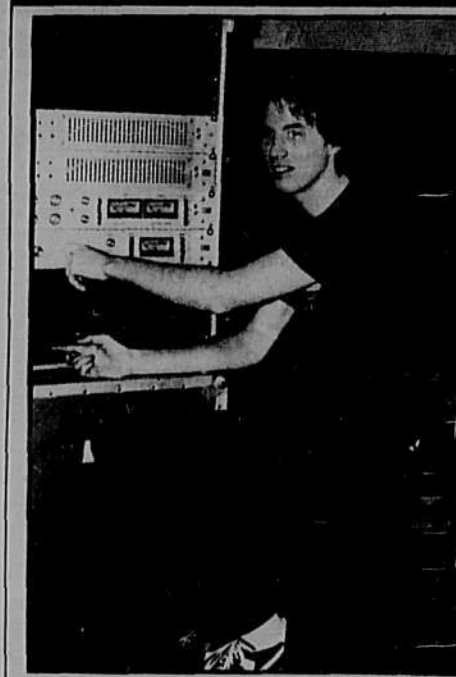
Audio-visual technician Lisa Simmons UPS System is not cost effective.
