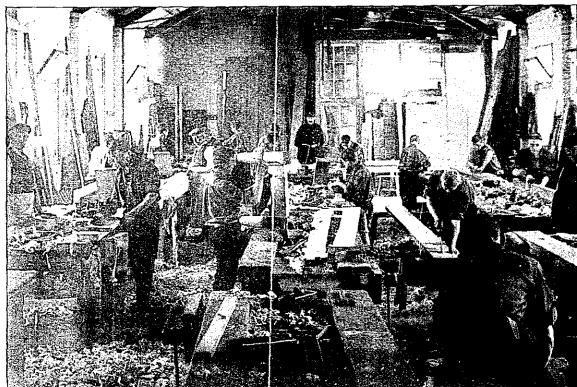
Carpentry, Borstal Institution, Borstal, England.
