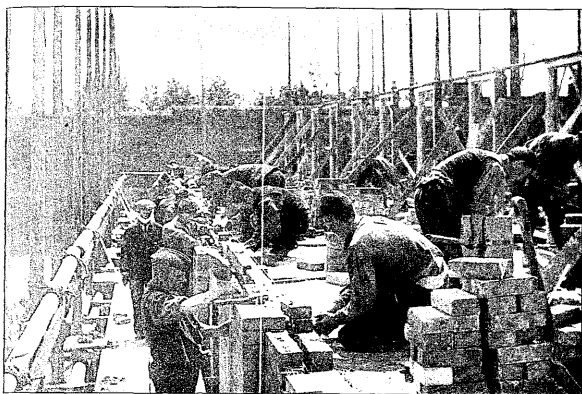
Building by Inmate Labor, Borstal Institution, Borstal, England
