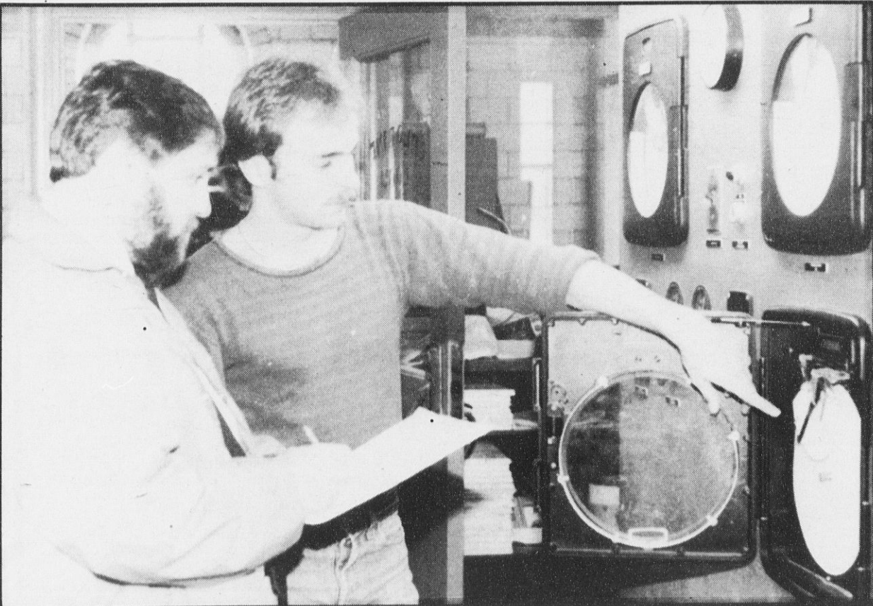
FILTER PLANT OPERATOR Robert Drosdowich shows Region III Field Representative Richard Blair one of the many meters that must be read accurately by filter plant employees in order to regulate the prison's water supply.
