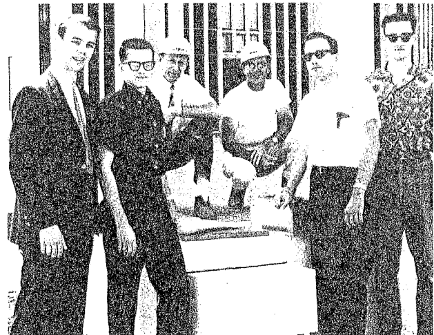
The laying of the cornerstone on Dutch Quad in 1964 included the burial of a time capsule by students.
