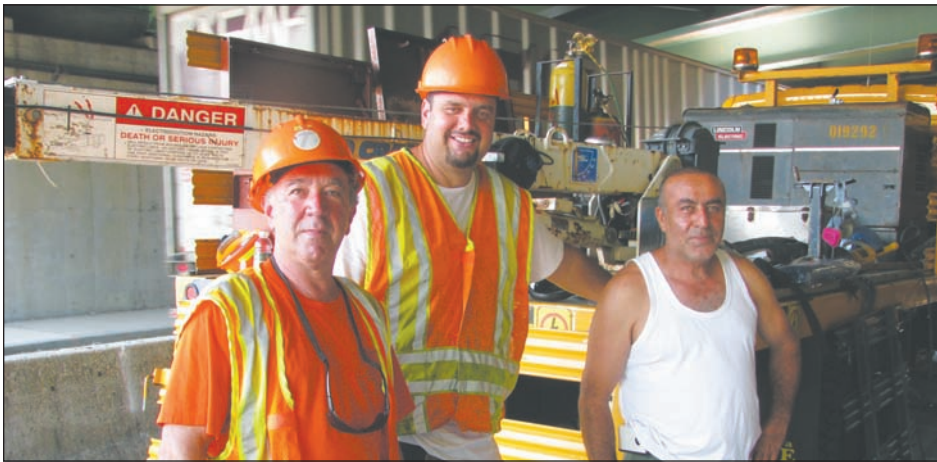
CSEA Long Island state Department of Transportation Local members Mike Cangiano, Philip Gaches and Yusut Izci were among those who made emergency repairs to a local overpass.
