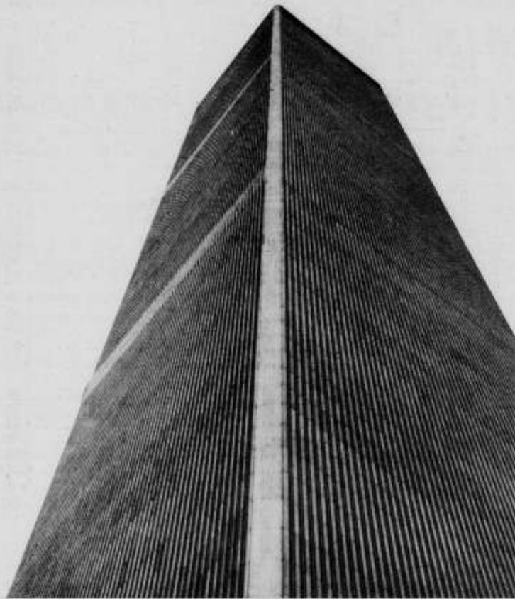
This is Building 2 of the World Trade Center, the 110-story twin giants in lower Manhattan. Although only 60 or so floors are occupied, the building is home to thousands of state employees.
