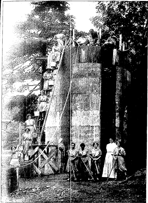
Construction at Bedford Reformatory
