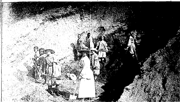
Ditch Work, Bedford Reformatory
